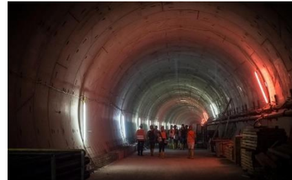
1-Subway Constructions in Karlsruhe
